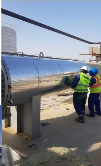
Pipes thermal insulation
