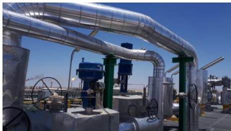
Pipes thermal insulation
